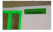
Heat Pump air handlers (also called "mini-splits") are placed in large areas to allow warm air to heat the rooms in the winter and to allow cold air to cool the rooms in the summer.
